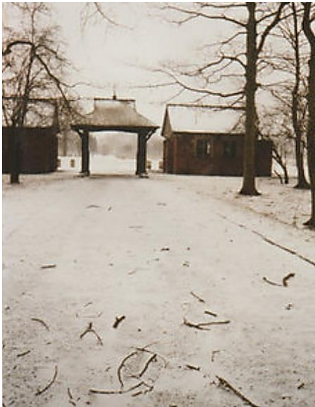
[above] Photograph taken in 1977/78 showing the route between point A and point B leading up to the lych gate
